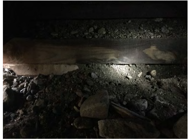
Right Bank Abutment when facing downstream
