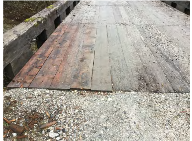
Some planks recently replaced at right approach
