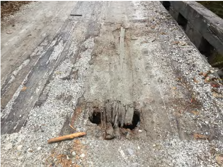
Timber deck condition
