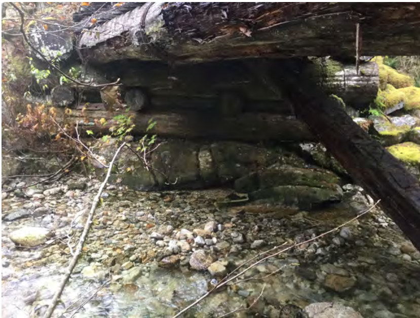
Right Abutment when facing downstream
