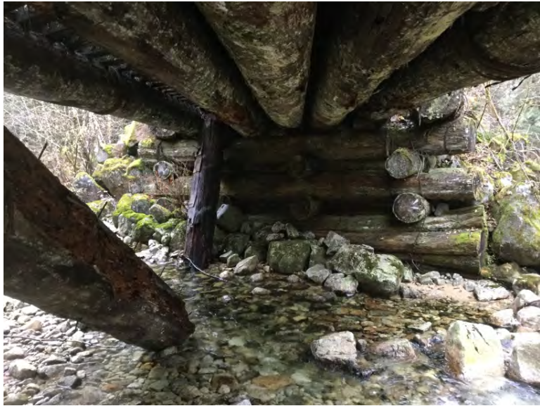
Left Bank Abutment when facing downstream
